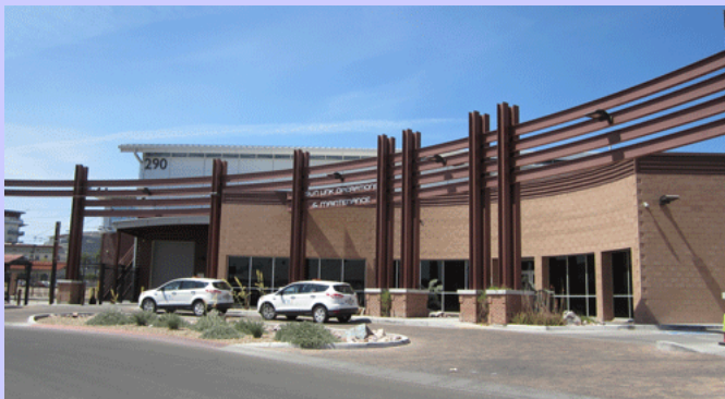
All eight of the cars are shown in the two-track yard with the maintenance facility shown in the background.
